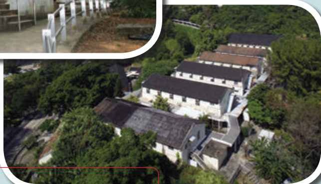
荔枝角醫院 (10)* Lai Chi Kok Hospital
